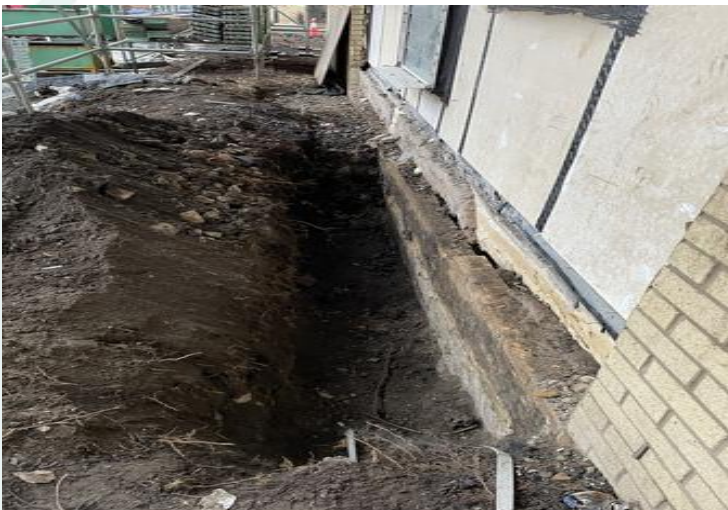
Blockwork foundation complete
